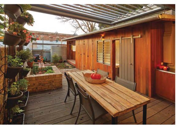
Leftover decking from the replacement of the balcony flooring lines the new exterior shed and seating area, while reclaimed sleepers are used for seating over the gabion walls, made from reused bricks from the demolished internal wall.
